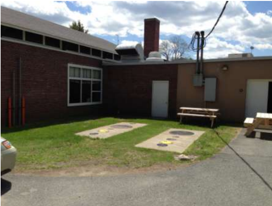
Figure 3. Exterior of Lyme School Boiler Room, oil tank locations seen in foreground
