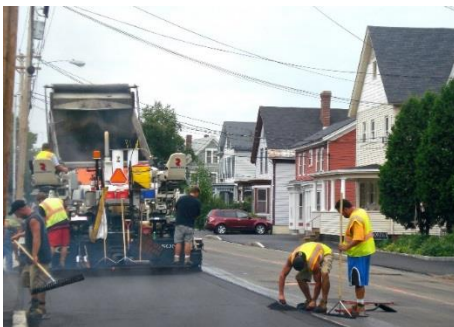
Road maintenance in Concord, NH. Credit:
