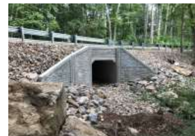
Culvert Replacement Barrington, NH
